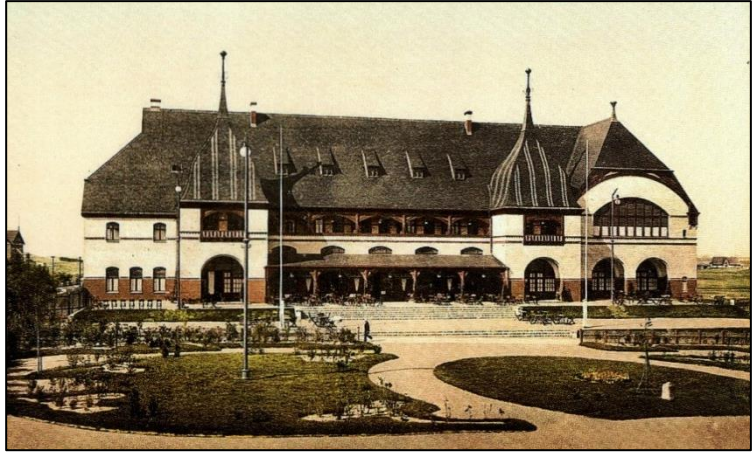
A picture of the large spa ( das Kurhaus ) in Westerland
